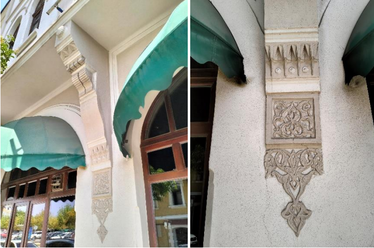
Figure 6. Consoles with overhangs on the side facades (Photograph: Eser Çalikuşu, 2023)
